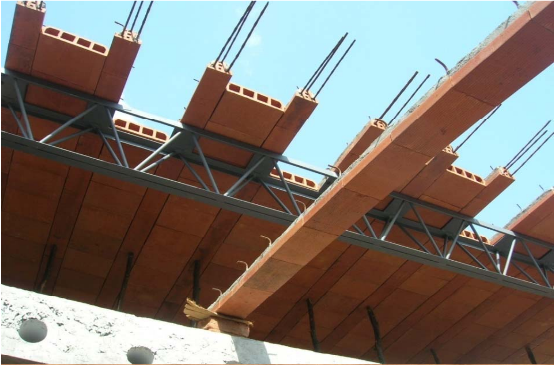
Roofing with terracotta hollow blocks
